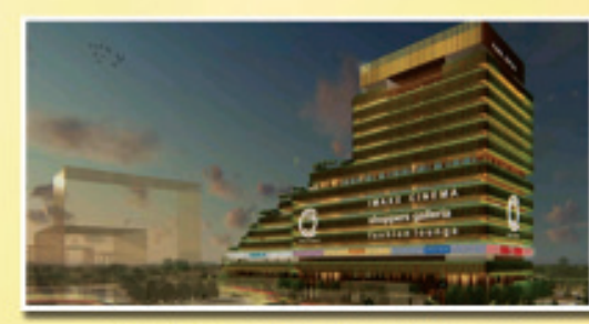
Multilevel Car Parking cum Commercial Complex at Agartala
